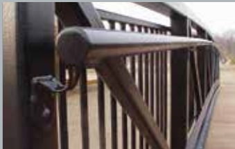
Vertical Picket/Pipe Handrail
